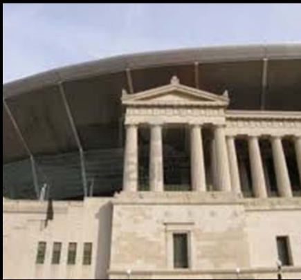
Architects destroy Soldier Field, Chicago
